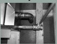
1. Close drain valve. (Skip this step with Auto Drain option.)
